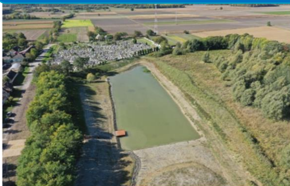
Multi-basin wetland to manage inland water inundation
